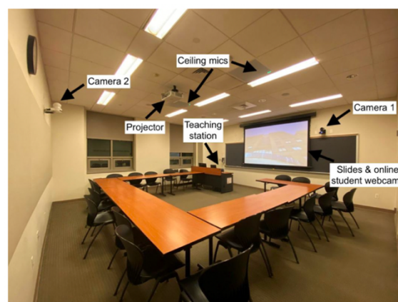
Figure 2. Example of HyFlex class setup and technology placement [12]
